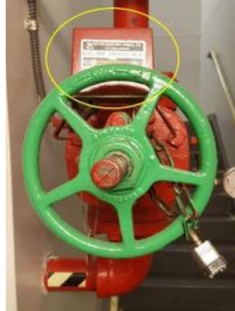
Tamper switch on a sprinkler valve
