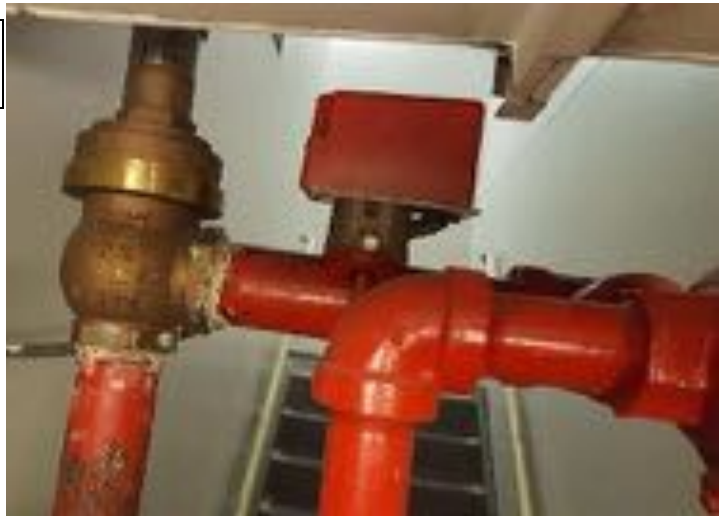
Water-flow Switch
