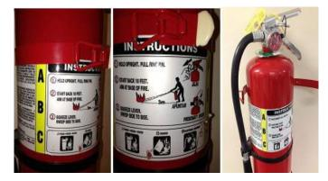
Class A portable fire extinguishers are available but are not as prevalent as Class ABC extinguishers. Class A portable fire extinguishers are also known as Air Pressurized Water (APW) fire extinguishers. Water is an extinguishing agent for regular combustibles.
