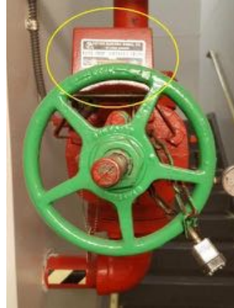
Tamper switch on a sprinkler valve
