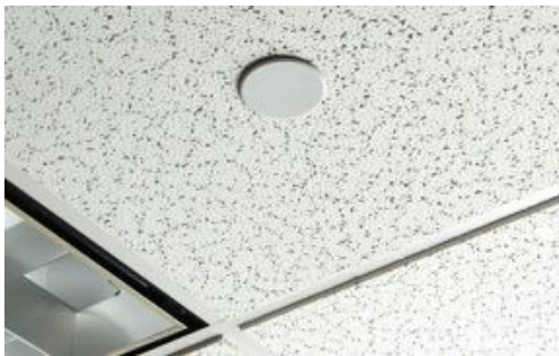
Concealed fire sprinkler heads with cover plates
